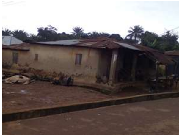
Figure 7. A single family apartment (Source: Authors field survey, 2016).
