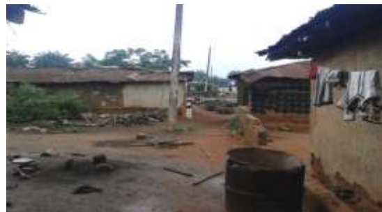
Figure 5. Building surrounding condition (Source: Authors Field Survey, 2016).
