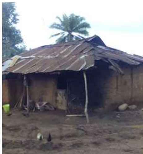
Figure 2. A single family apartment (Source: Authors field survey, 2016).
